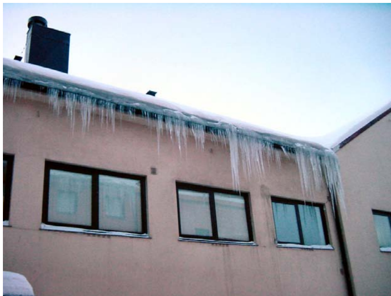
Figure 1. Building with icicles and icing on the overhang.
